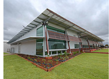
The new McWilliam's Wines administration and laboratory building is a skillion roofed single level structure clad in LYSAGHT CUSTOM ORB® and LYSAGHT SPANDEK® profiles made from ZINCALUME® steel.
